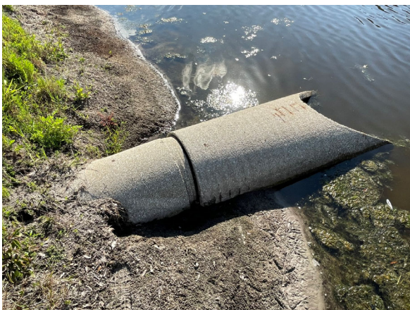
Partially separated 18" MES at Pond A2
