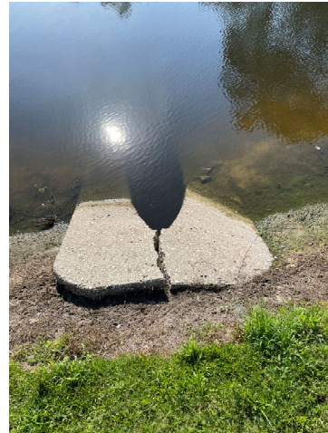
Moderately Cracked 24" MES at Pond T2
