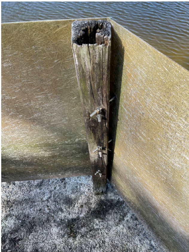
Deteriorating wood at Pond T2 weir outfall
