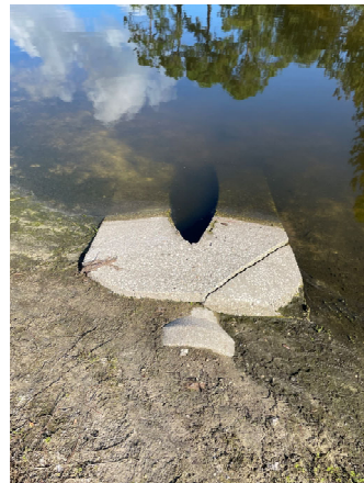
Minor crack in 18" MES at Pond T2
